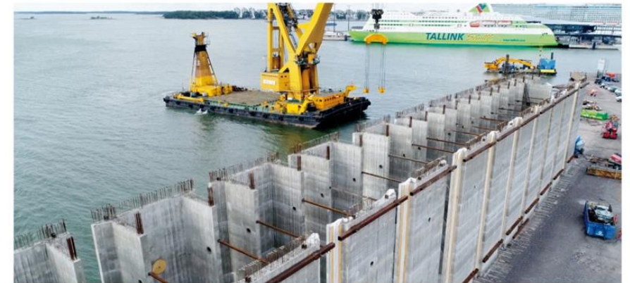
QUAY WALL PROJECTS
